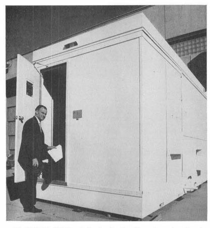
ALL-WEATHER MODEL of the Sandia Ultra-Clean Room is pictured with designer Willis J. Whitfield (2564-2). Even in New Mexico sand storms, the unique air flow and absolute filter features have provided a work area free of microscopic dust particles. Room is easily moved.
